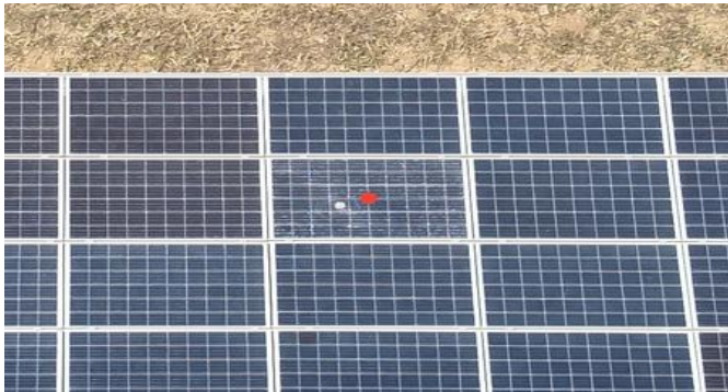
DJI_20230719112118_0951_V.JPG DJI Mavic 3T Enterprise
