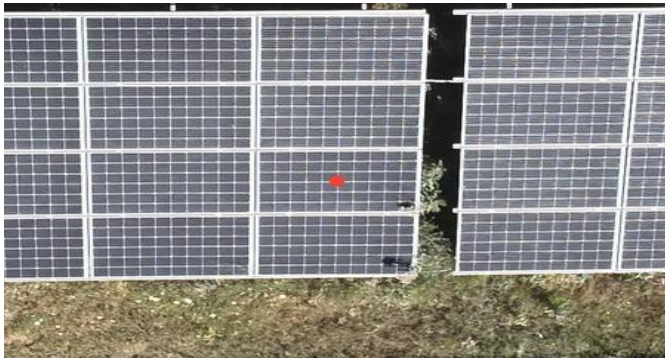
DJI_20230719114723_0538_V.JPG DJI Mavic 3T Enterprise
