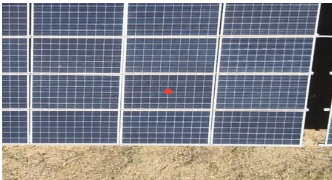
DJI_20230719111852_0821_V.JPG DJI Mavic 3T Enterprise
