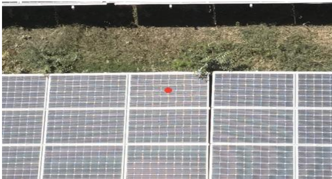
DJI_20230719114923_0646_V.JPG DJI Mavic 3T Enterprise
