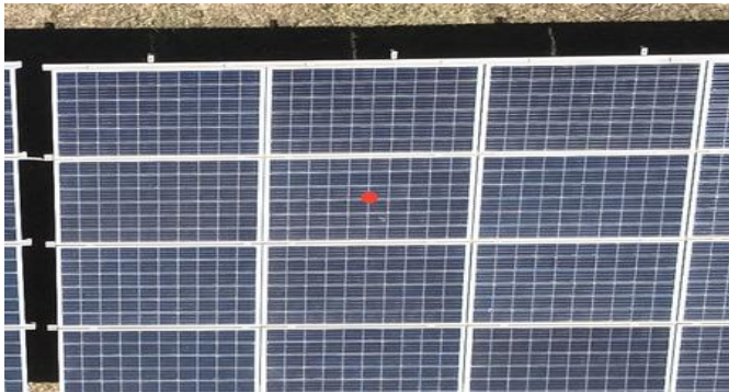
DJI_20230719112110_0944_V.JPG DJI Mavic 3T Enterprise
